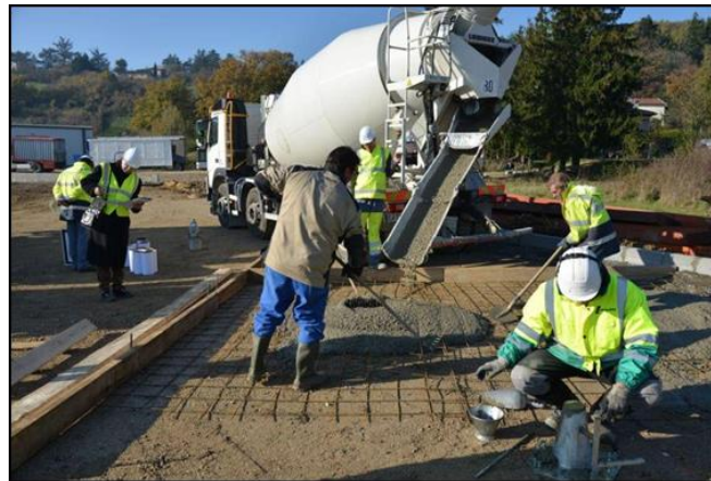
Car-park experimental demonstration site Recycled aggregate rates: 0, 30 and 100%
