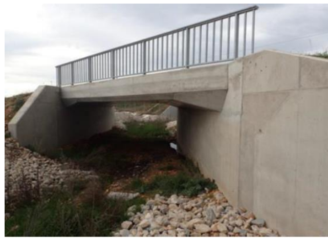
Bicycle bridge demonstration site Recycled aggregate rate: 20 % (40% also tested in lab)
