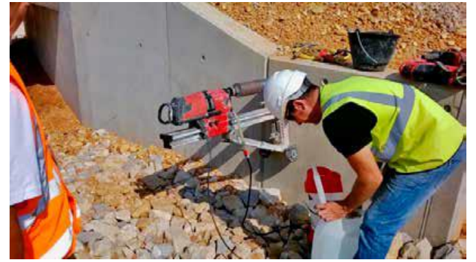
Core sampling in testing wall
